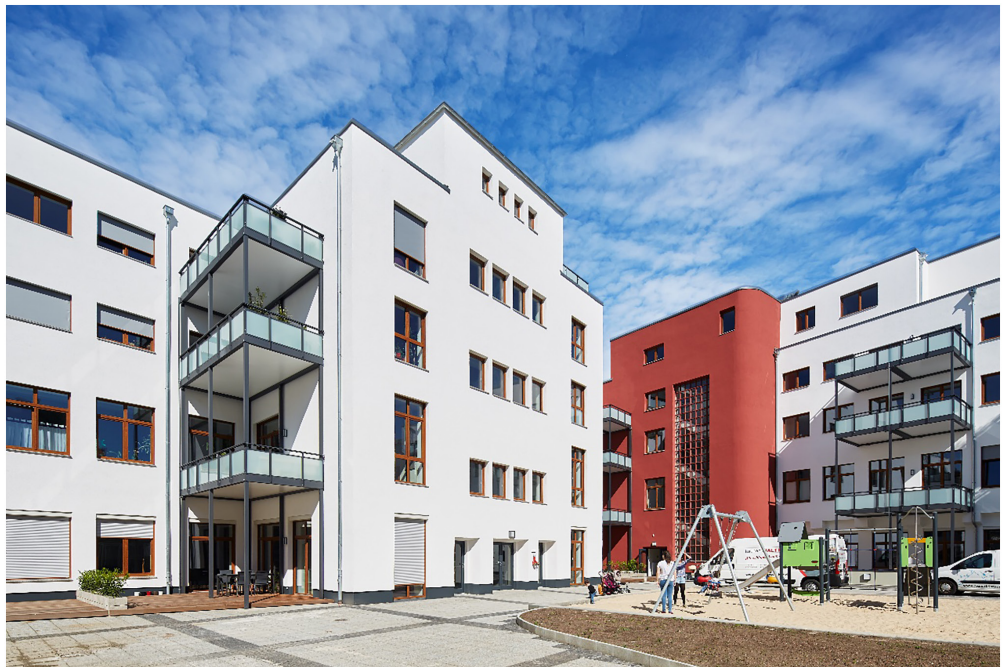
Figure 3 A former production facility for bicycles, mopeds, and typewriters, which had already been converted into office space in the 1990s, was redeveloped into 88 apartments and two commercial units (Photo credit: Knauf/Sigi Lustenberger)
