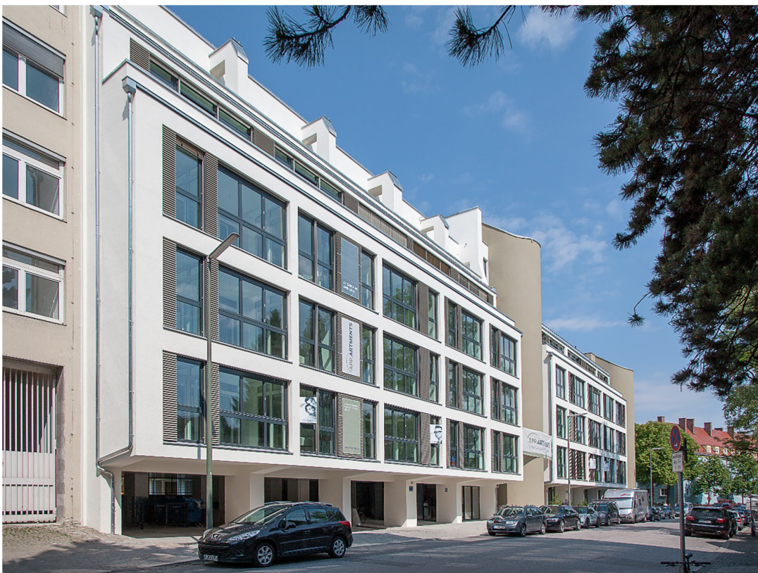
Figure 1 A former insurance administration building was converted into 167 apartments (Photo credit: Knauf/Bernd Dücke)
