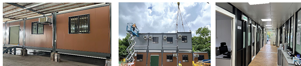
Assembly of module and internal finish
