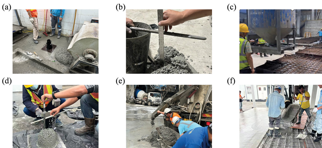
Figure 4 Photographic documentation of HPLWC production: (a) lab trial, (b) plant trial, and (c) full-scale production for the first project; (d) lab trial, (e) plant trial, and (f) full-scale production for the second project
