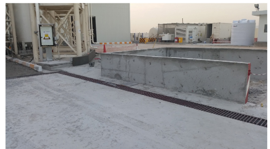
Figure 2 Use of low carbon concrete on aggressive industrial environment
