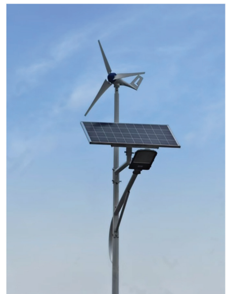
Figure 2 Solar and Wind Powered Intelligent Lighting System
