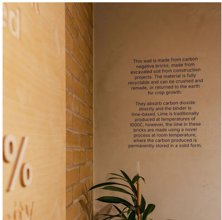
Figure 3 The “Wonderwall” pilot project in Manchester: a 4 x 4 m wall clad with N10 bricks, working as a carbon-sink and able to absorb a total of 213 kg of CO 2 over its life cycle. The wall is constructed in collaboration with the company Sustainable Ventures and serves as a public proof of concept of the technology. The 1200 bricks wall is estimated to sequester 213 kg of CO 2 over its lifespan. The wall will continually draw CO 2 from the ambient air and permanently store it as calcium carbonate within the masonry. This pilot project showcased the bricks’ structural viability and aesthetic (the earth-tone bricks have natural, variegated colors without any pigmentation) as well as their environmental potency, as the wall will act as an active carbon sink over its lifecycle. The project underscored that even a small structure built with e4E materials can offset emissions—in this case, equivalent to the CO 2 emitted from making ~760 cups of coffee
