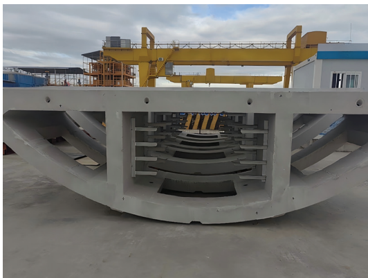
7 Precast tunnel units waiting for construction
