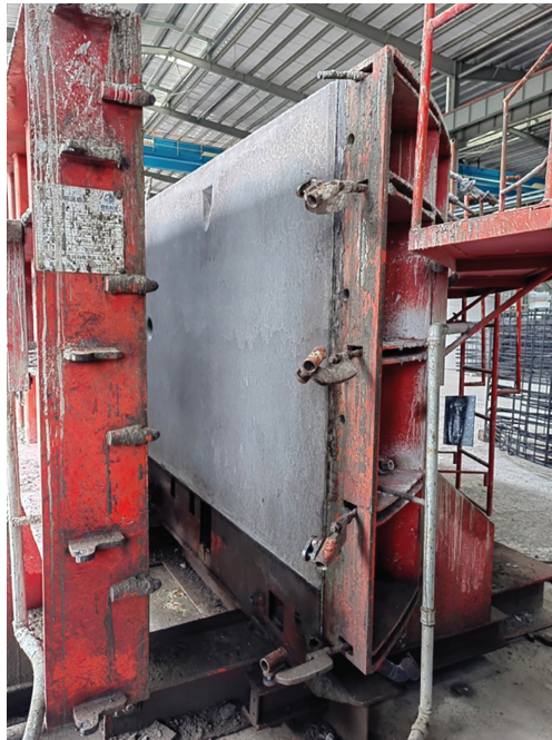
5 Precast tunnel unit demolding
