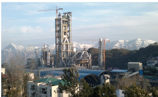
1 Photo: Darlaghat-Rauri Cement Plant, located in Himachal Pradesh (Credit: Ambuja Cements)
