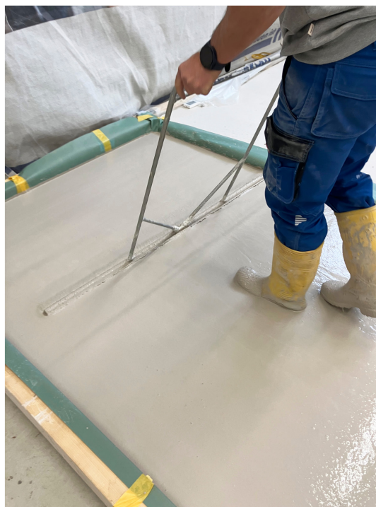
13 Process of equalizing screed
