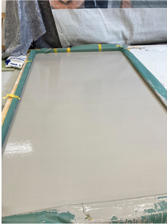
14 Screed surface after completion
