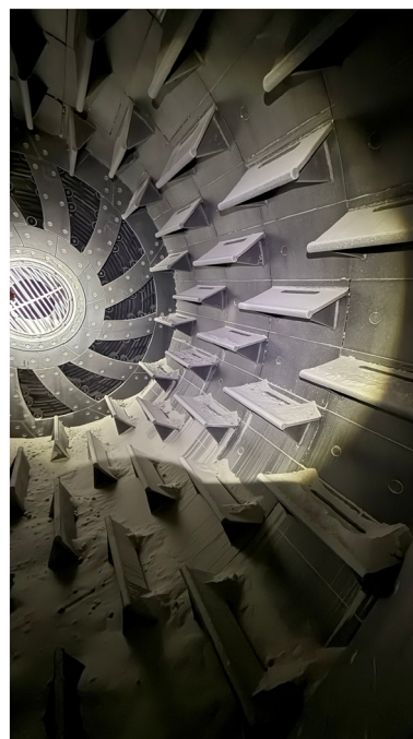
5 Drying Chamber Elements Installed
