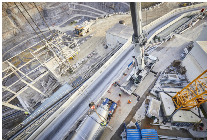
The Hahnstätten lime plant includes a new packing complex
