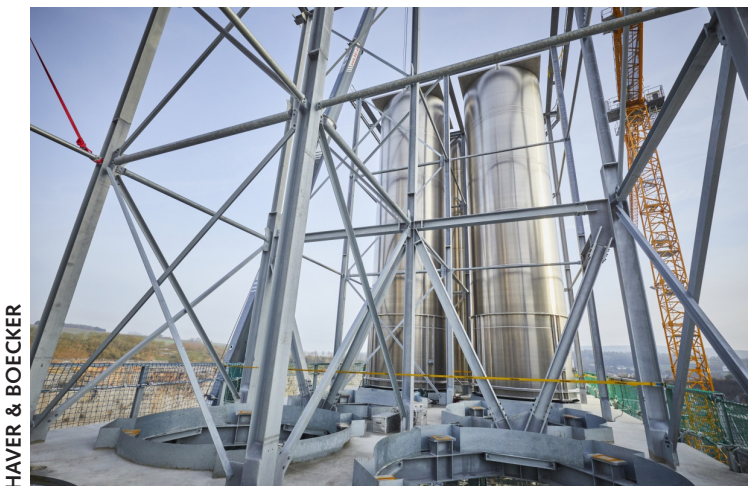
In the silos, the PCC will be deaerated by sedimentation and fed from there into three HAVER & BOECKER packers, depending on requirements and customer applications
